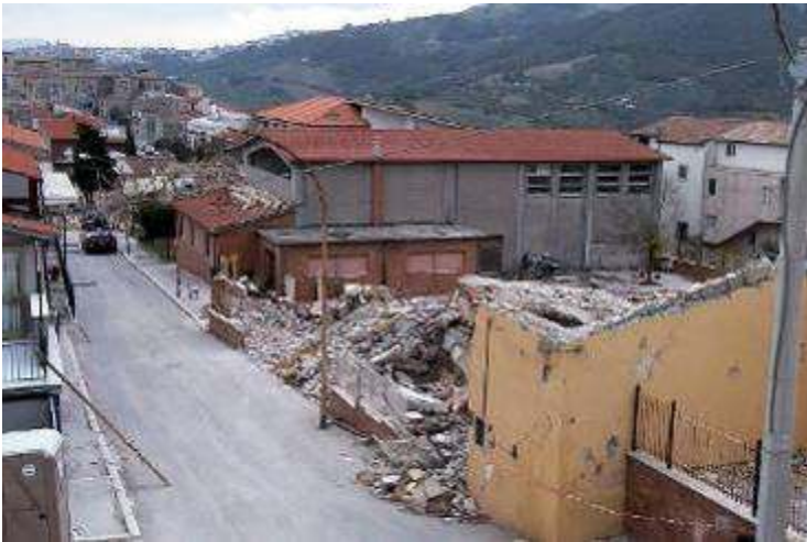
Figure 1.26. The school in San Giuliano di Puglia that collapsed during the Molise 2002 earthquake, causing the death of 27 pupils and one teacher.
